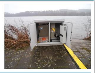
The BACTcontrol detects the presence of bacteria - including E.Coli and coliforms - in water. The online monitoring is based on an Enzymatic reaction that makes the bacteria visible for fluorescence detection.
